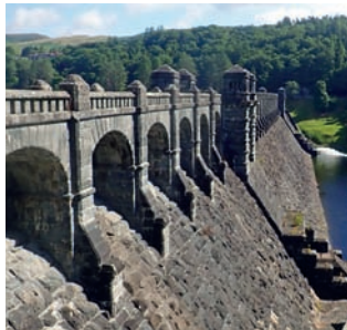
Above and below: Lake Vyrnwy with its stone dam wall and iconic tower was built in the 1880s to supply Liverpool with clean water.
